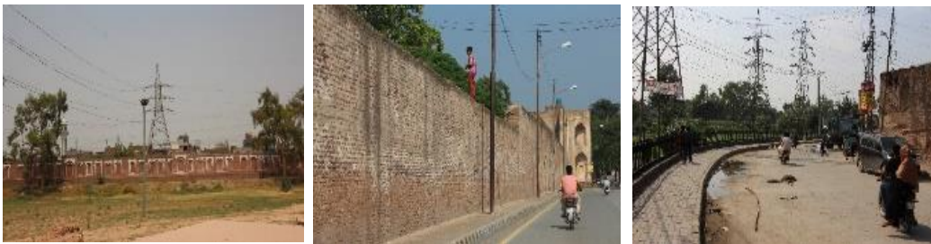
Figure 10 Electrical Infrastructure which is glued and overshadowing Shahdara Monuments. Source Author
