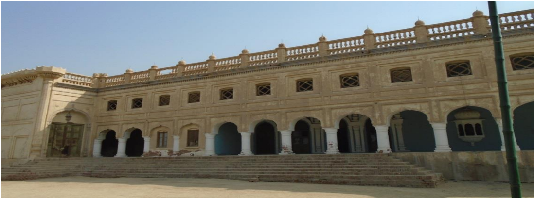
Fig#4 Portal view from northern side
