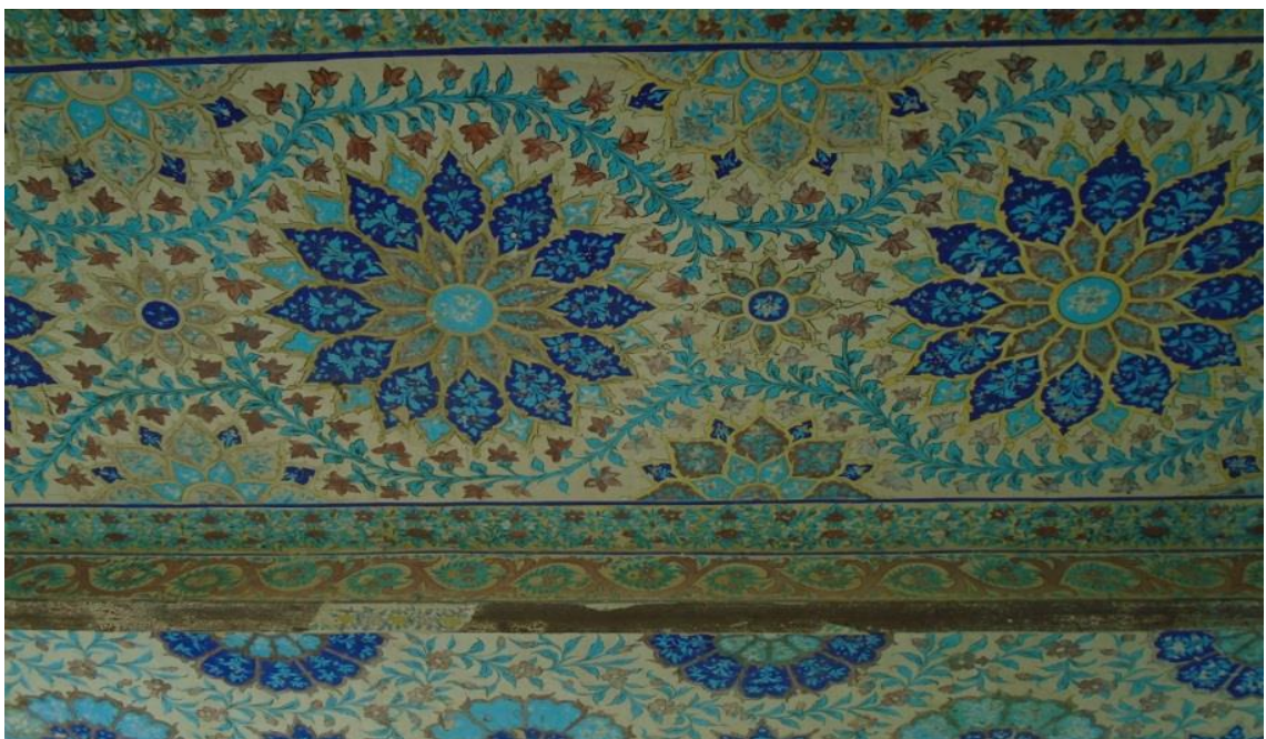
Fig#7. the ceiling decoration of southern veranda
