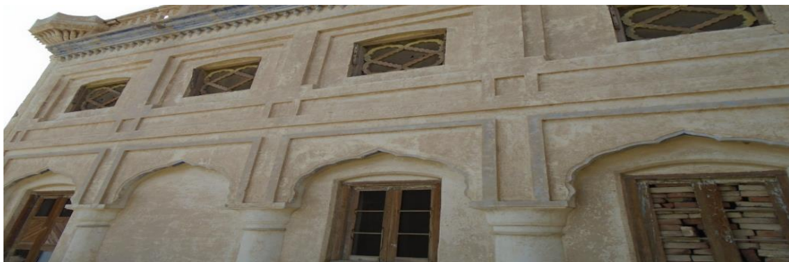
Fig#3 Exterior view of facade of the building
