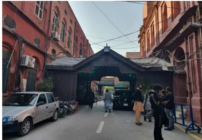
Figure 8: View of Entrance lobby to the offices behind Jinnah Hall
