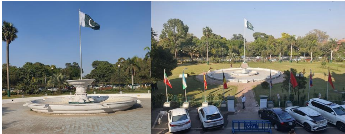
Figure 6 : View of Foundation and Garden in front of Town Hall
