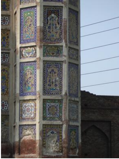
Figure 8. Semi-attached octagonal minaret with faience mosaic panel and remnants of boundary walls behind. (Picture by Author)
