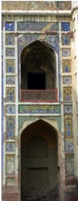
Figure 7. Double-storied arches flanking the central three-centered arch on the façade facing the east. (Source: Picture by author)
