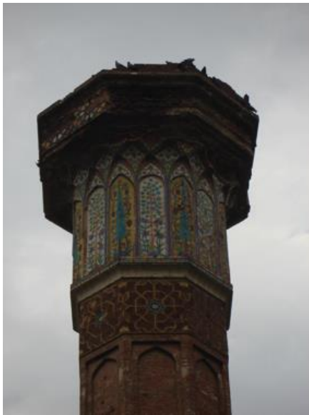
Figure 9. Chauburji tower crowning structure with faience mosaic and cut-brick work underneath. (Picture by Author)
