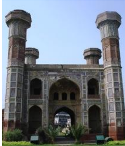
Figure 1. Main façade of Chauburji gateway of 1646 at Lahore facing east
